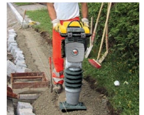
Exact unit guiding – important during compaction in border areas.
